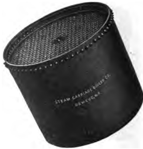
FIG. 402.—Bottom View of a Type of Boiler shown in Fig. 145, exhibiting the method of riveting in the lower tube plate.
