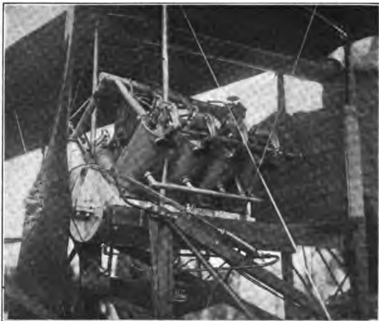
FIG. 415.—Outlining installation of power plant in Curtiss biplane.
