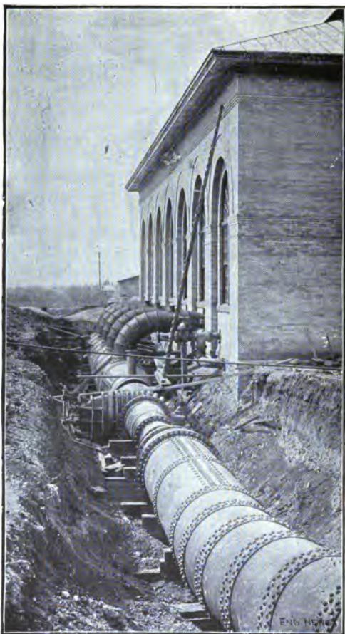
FIG. 75 i .—THE VENTURI METER IN POWER STATION.
