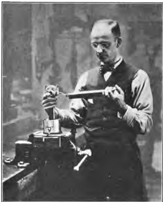
FIG. 63.—Fitting piston pin.
